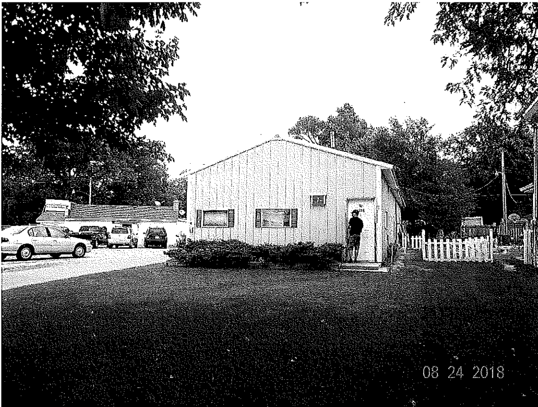
P4. Looking easterly from the Benton Street and the southwest corner of the site.
