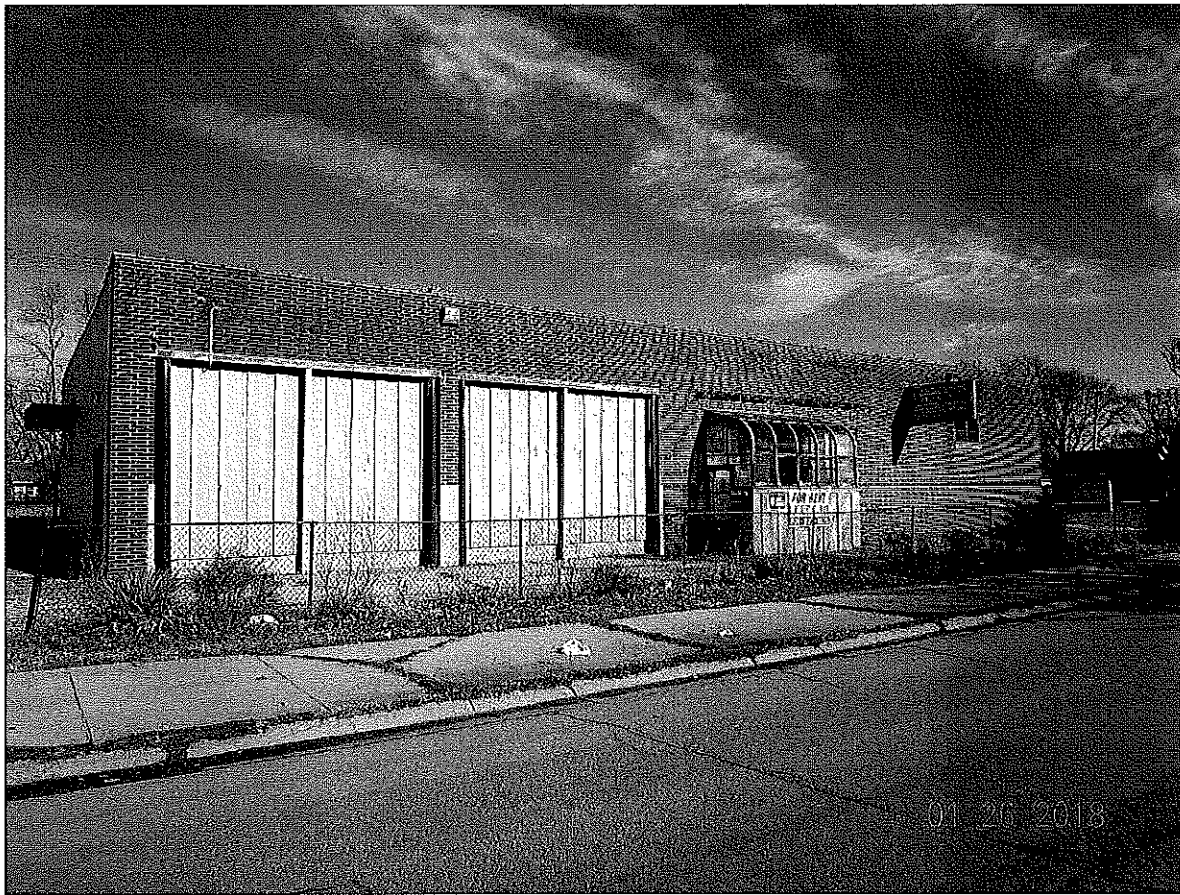
P2. Looking northerly toward the front of the building from W. 6 th Street.
