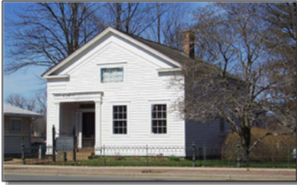
Award for Adaptive Reuse Dr Glenn Wheel 900 Lincolnway West Ellis Schindler House Greek Revival c.1834 Outstanding #46005
