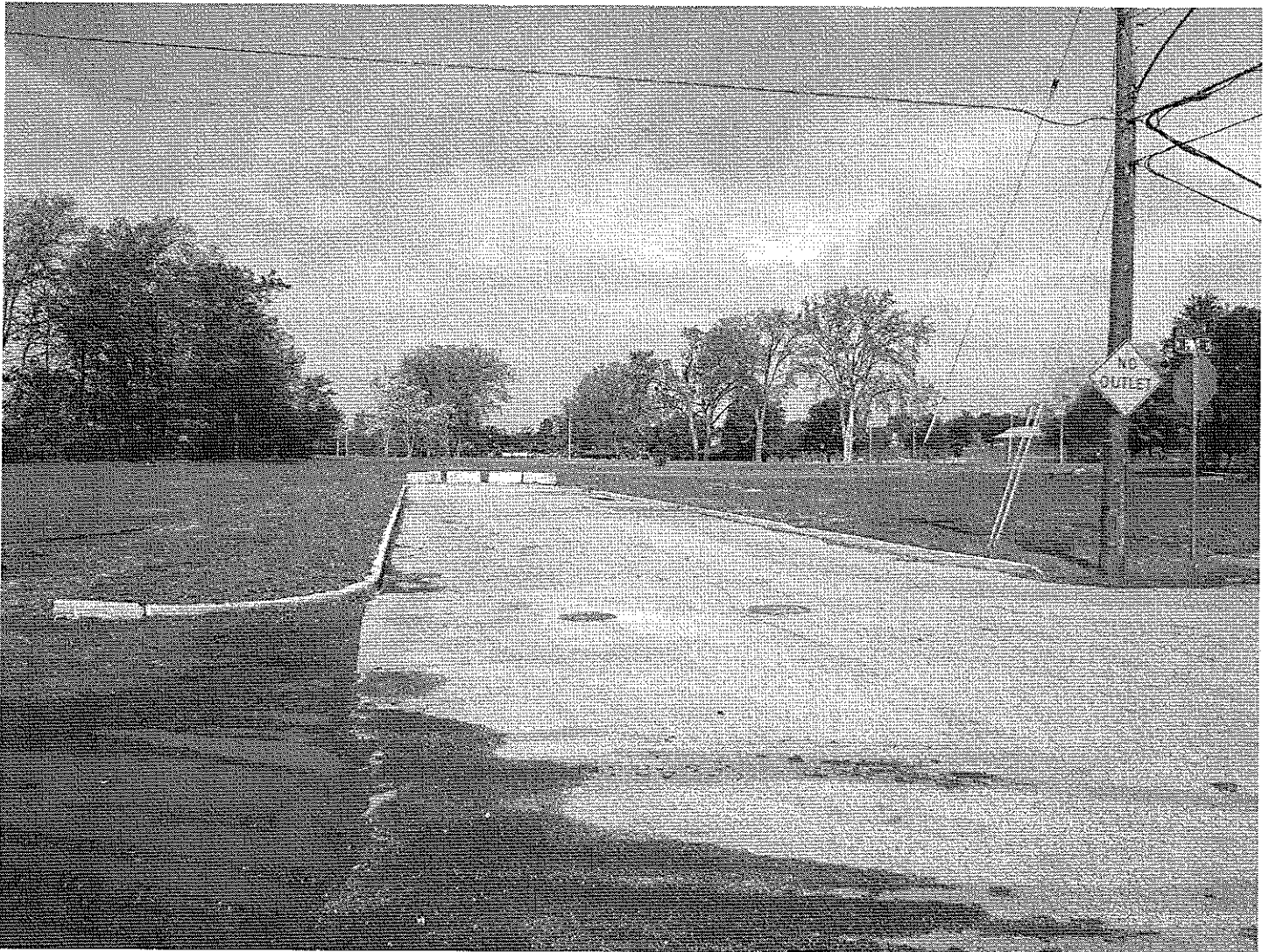
View looking onto Madison Street to be vacated
